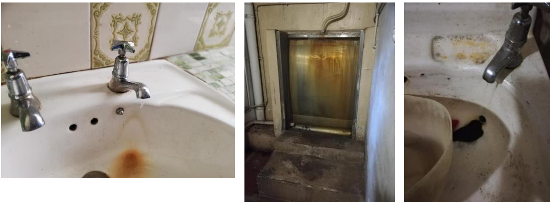
Figure 20: Leaking taps and fittings shown to be a long-term problem, as illustrated by stains in the basins and urinal in the basement.
